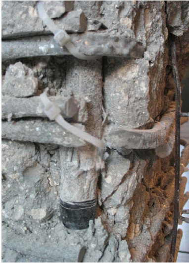
Figure 16– Bar B 3-inche tie spacing: failure detail
