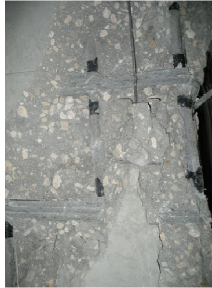
Figure 18 – Bar B 12-inch tie spacing: failure detail
