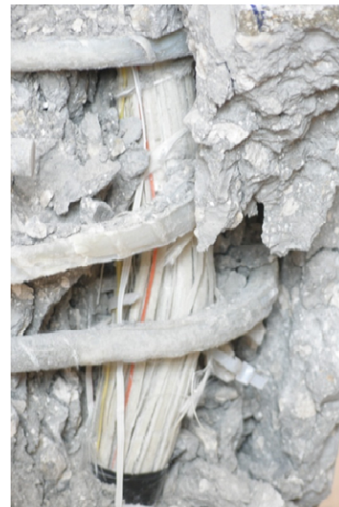
Figure 15 – Bar A 3-inche tie spacing: failure detail
