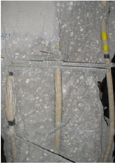
Figure 17 – Bar A 12-inch tie spacing: failure detail
