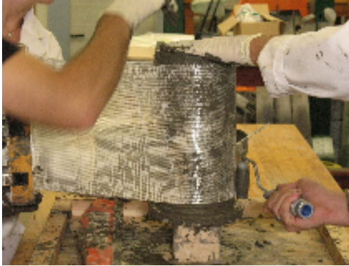
Figure 6 - Embedding fiber with ribbed roller.
