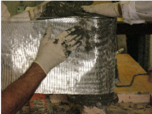
Figure 7 - Application of grout.
