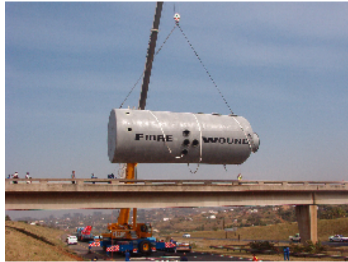
Figure 5: Photograph of FRP Scrubber Vessel in transit to site. (Zone 3)
