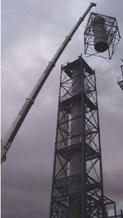
Figure 6: Photograph of FRP stack module being assembled (Zone 5)
