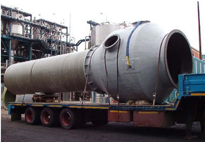
Figure 2: Photograph of Gas Inlet Ducting (Zone 1)
