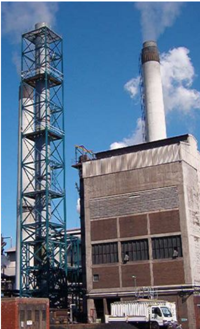
Figure 6: Photograph of FRP stack module being assembled (Zone 5)
