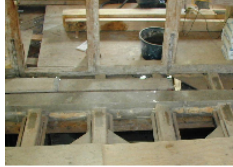
Figure 6: PC reinforcement from upper floor
