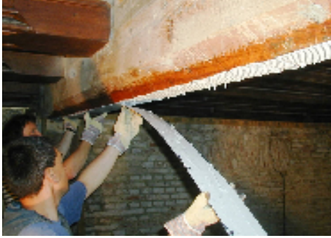
Figure 5: Gluing of the FRP strips
