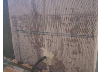
Figure 4: Panel in vacuuming stage
